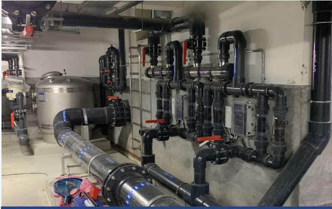
MECHANICAL, ELECTRICAL & PLUMBING INSTALLATION
